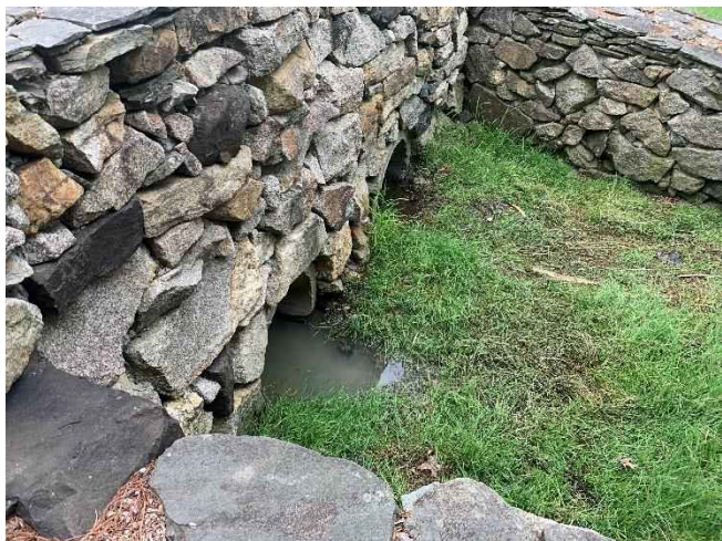
4 Brickyard Circle - 1 (Drainage Course)
