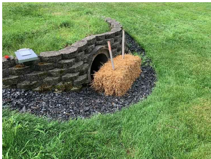
29 Gundalow -1 (Drainage Area)
