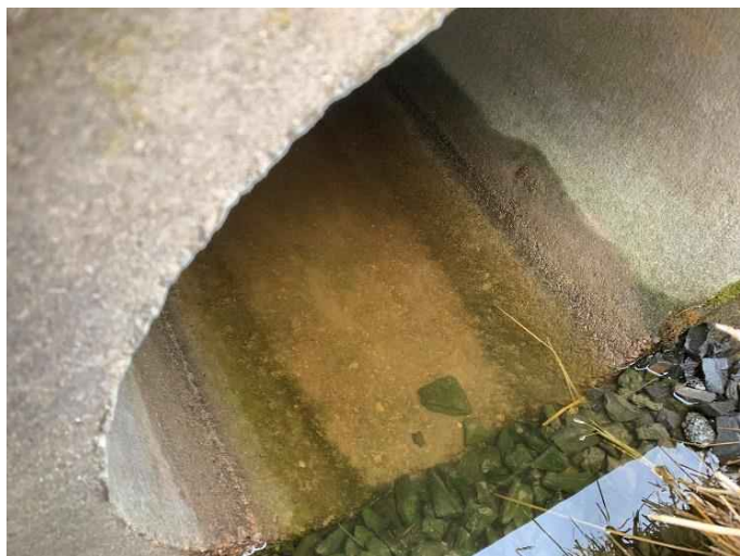
29 Gundalow -1 (Drainage Area)
