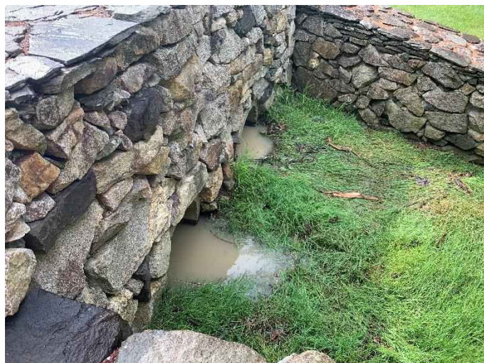
4 Brickyard Circle – 1 (Drainage Course)
