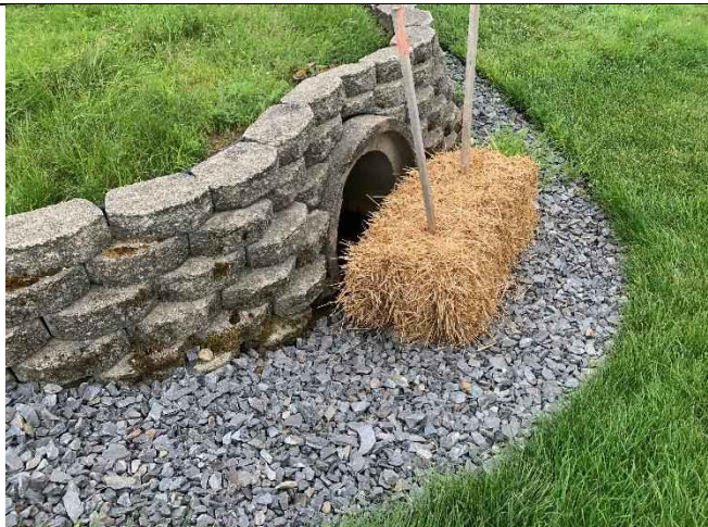
29 Gundalow - 1 (Drainage Area)
