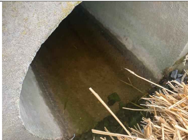
29 Gundalow - 1 (Drainage Area)
